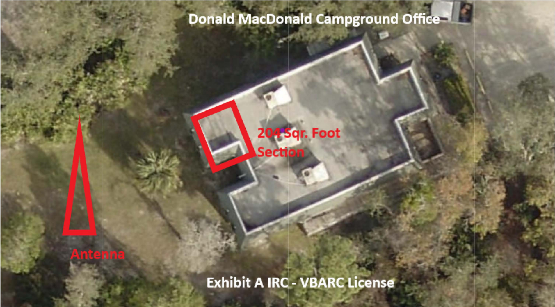
Donald MacDonald Campground Office - Exhibit A
