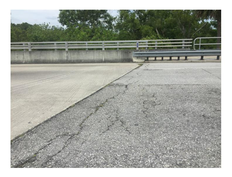
Infiltration of water through endwall diaphragm.
