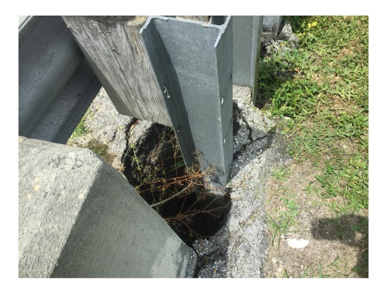
Undermining of guardrail and loss of miscellaneous asphalt.
