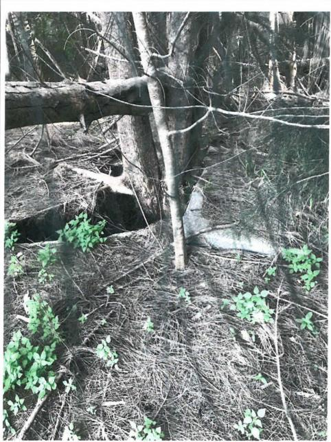
2/6/18 4:21pm Photo 1 Tree growing out of broken septic tank behind Structure A(Church)
