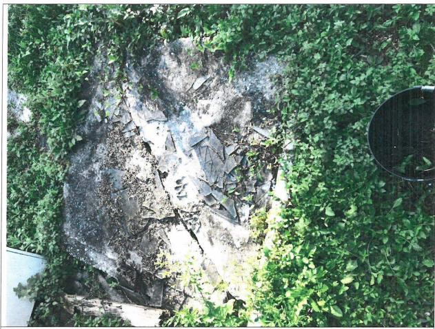
2/6/18 4:05 Photo 5 Broken Septic Tank serving structure C(Duplex 1)
