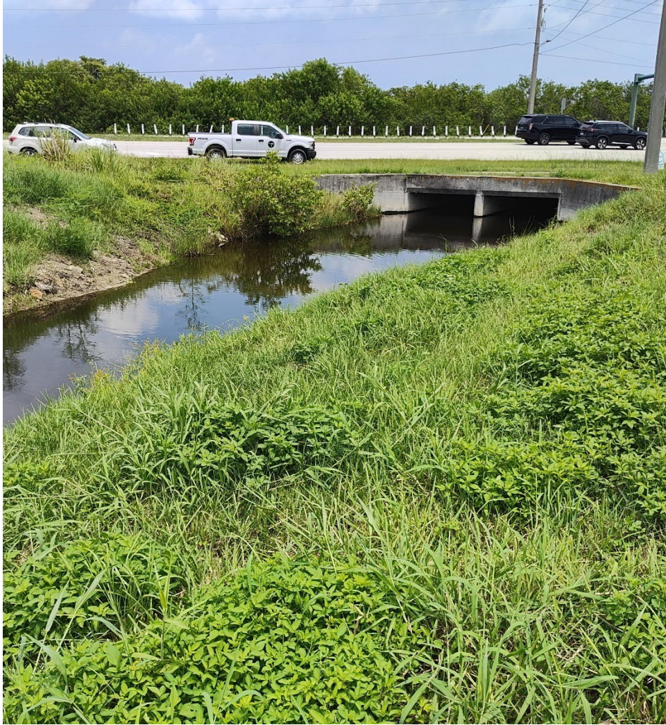
Figure 14. Ditch with Water and Box Culvert facing East along 37th Street. Photo #1.
