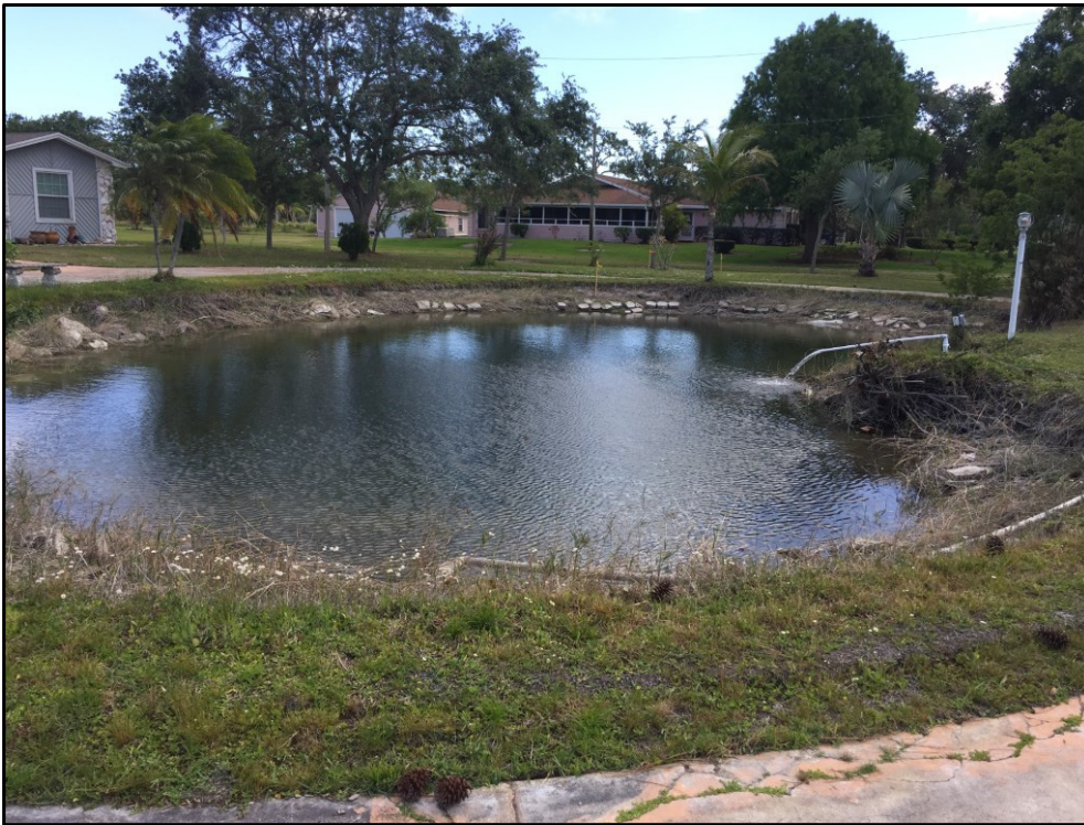
POND VIEW FRONT VIEW
