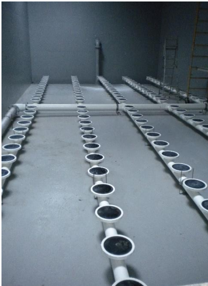
Figure 1 - When the tank was initially constructed in 2010
