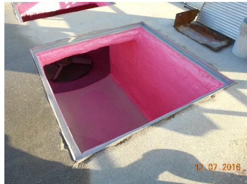
Figure 1-After SpectraShield Liner System was installed at Central WWTP
