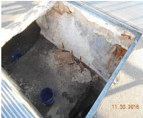
Figure 2- Before SpectraShield Liner System was installed at Central WWTP
