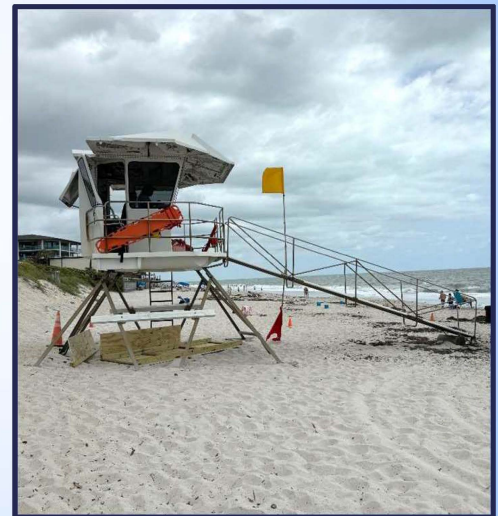
Current temporary station
