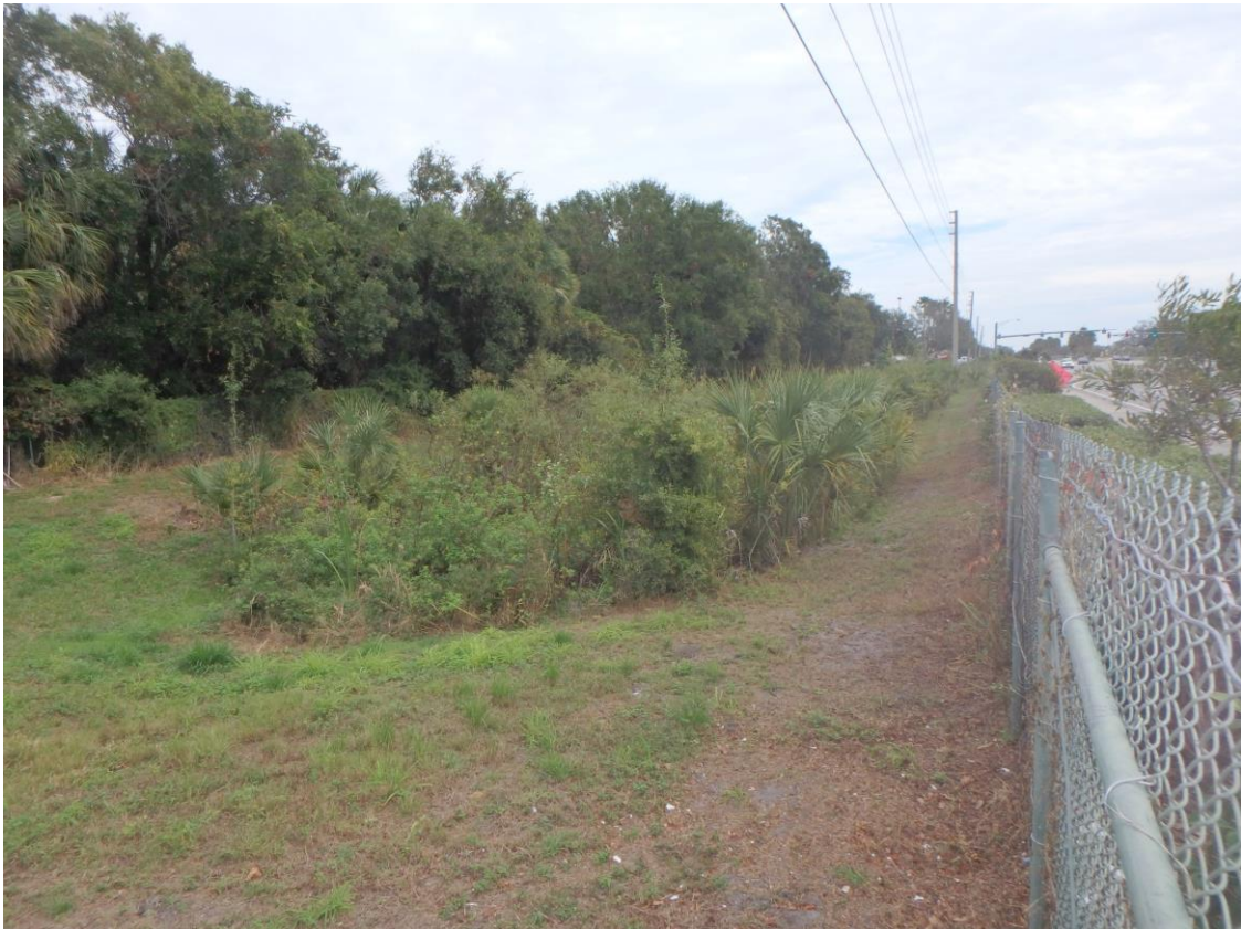
Photos of stormwater pond along SR 60, southern edge of property
