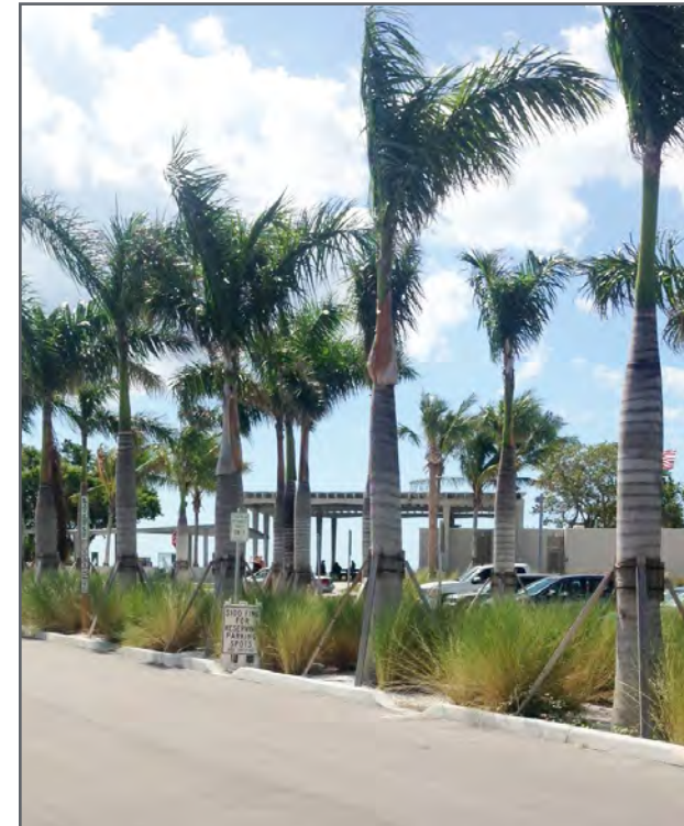
Bioswales are a Low Impact Development practice that utilize native plants to improve water percolation and remove pollutants.
