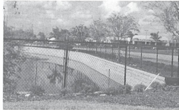
Photo Exhibit 1.1.16a Pond slopes and maintenance easements are preferred to avoid pond fencing.
