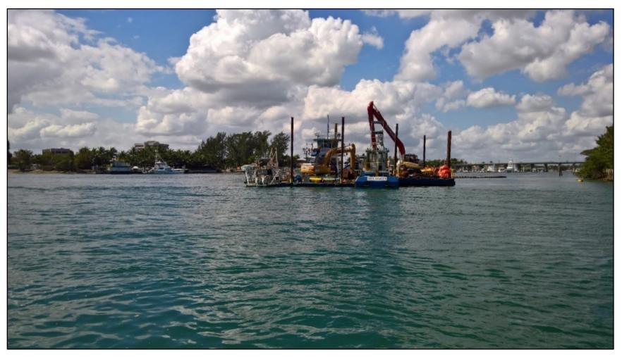
**Figure 13:** Jupiter Inlet with the Cavache Dredge working within the inlet to bypass sand, March 2017. Photo by Libbie McDearmid (DEP) in March 2017.
