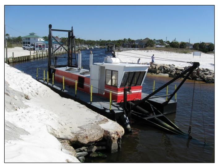
**Figure 21:** Mexico Beach Inlet being dredged to bypass material to Mexico Beach, photo by Ralph Clark (DEP) in April 2010.
