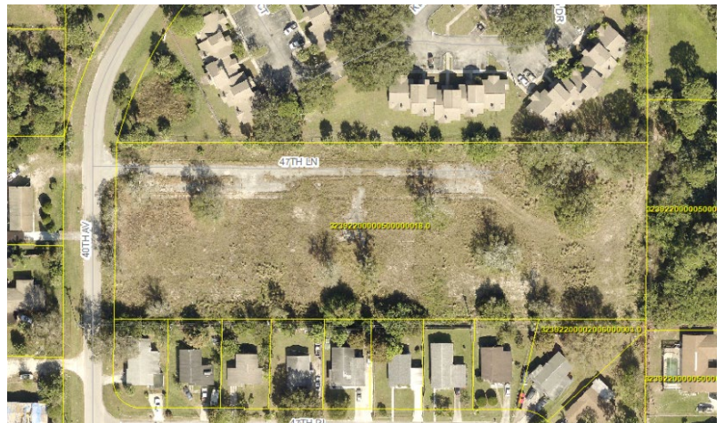
Aerial Photo, Former Gifford Gardens Site
